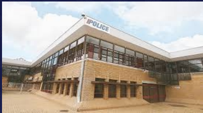
Henderson Police Station
